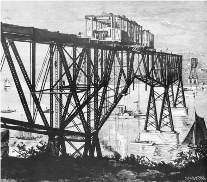
Poughkeepsie Bridge over the Hudson, New York, by Charles Macdonald and A B Paine, 1886-8. Completion of one of the main spans: Scientific American , 4 February 1888, no page.
