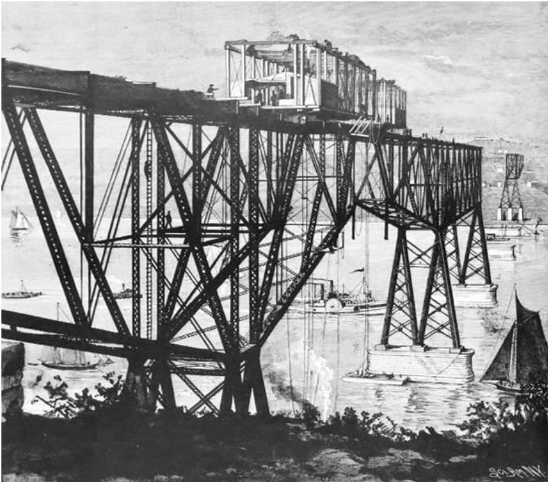
Poughkeepsie Bridge over the Hudson, New York, by Charles Macdonald and A B Paine, 1886-8. Completion of one of the main spans: Scientific American , 4 February 1888, no page.
